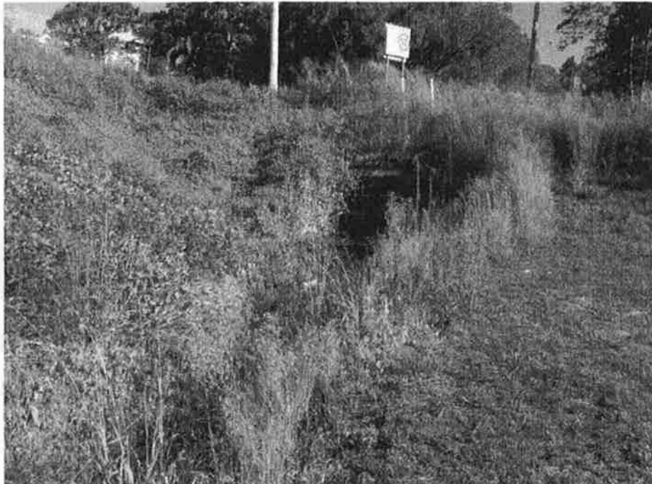
Plate 1: North view long drainage line toward Oban Street
